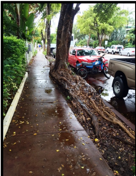
Concrete cut – sidewalk narrowed.
